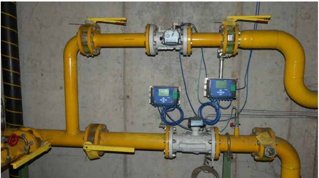
Zähler Methangas Contatori gas metano
